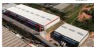
SPT Business Park 28.000 m 2
